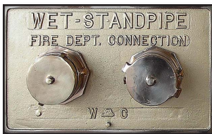
Figure 11-20 Automatic-Wet Standpipe Connection
