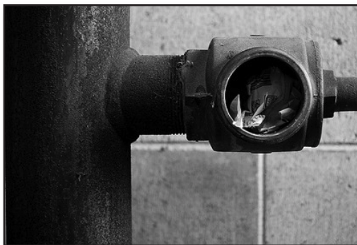
Figure 11-25 Standpipe Obstruction
