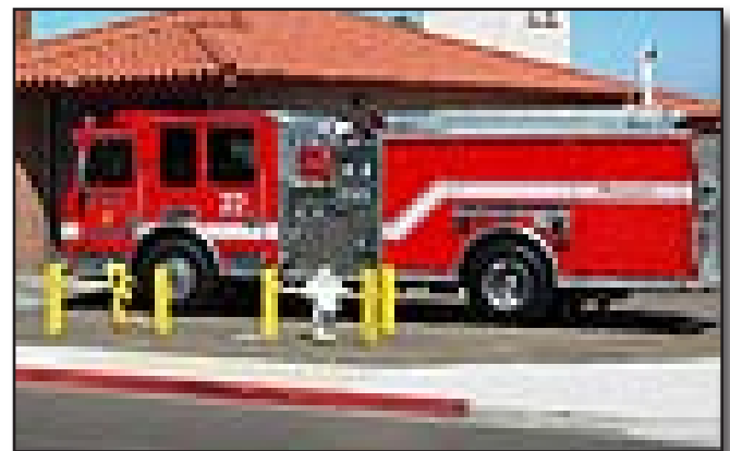
Figure 11-7 High Volume / Low Pressure Fire Hydrant
