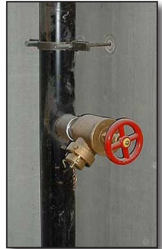
Figure 11-17 Class I Standpipe System
