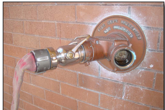
Figure 11-22 2 1/2" Hoseline Connected to the FDC
