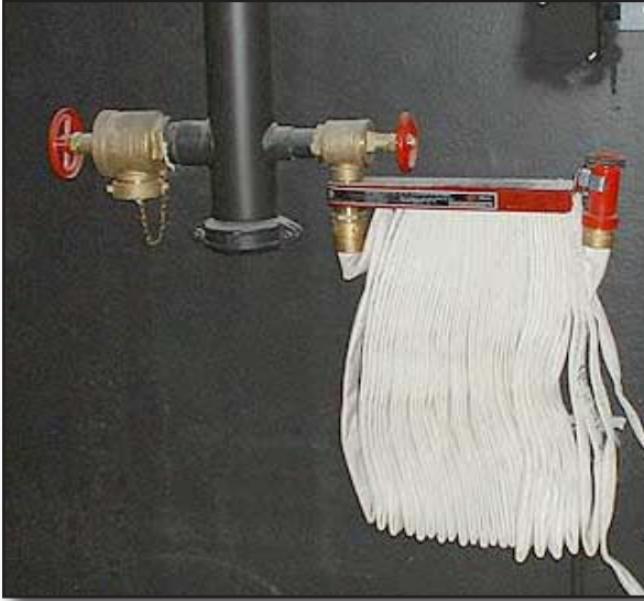
Figure 11-19 Class III Standpipe System
