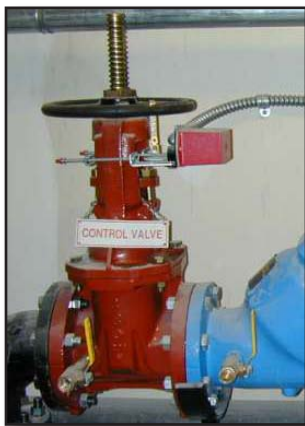
Figure 11-36 Outside Stem & Yoke Valve (OS&Y)
