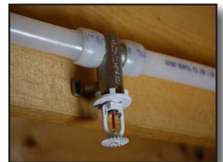
Figure 11-34 CPVC Sprinkler System Pipe
