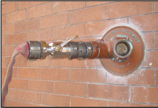
Figure 11-23 Double Female & Male Adaptor to FDC
