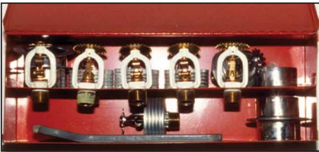
Figure 11-46 On-Site Sprinkler Head Replacements
