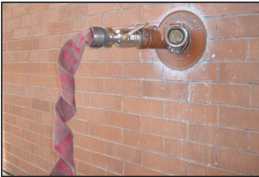
Figure 11-24 Twisting Hose to Connect to FDC
