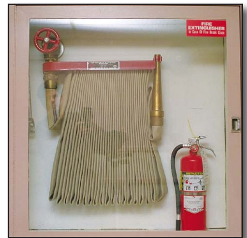
Figure 11-18 Class II Standpipe System
